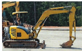
Road Base & Sub Base Stabilization
